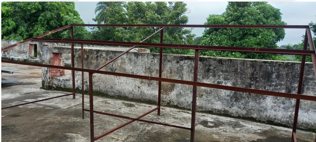
The structure for Future plan for installation of solar panels
