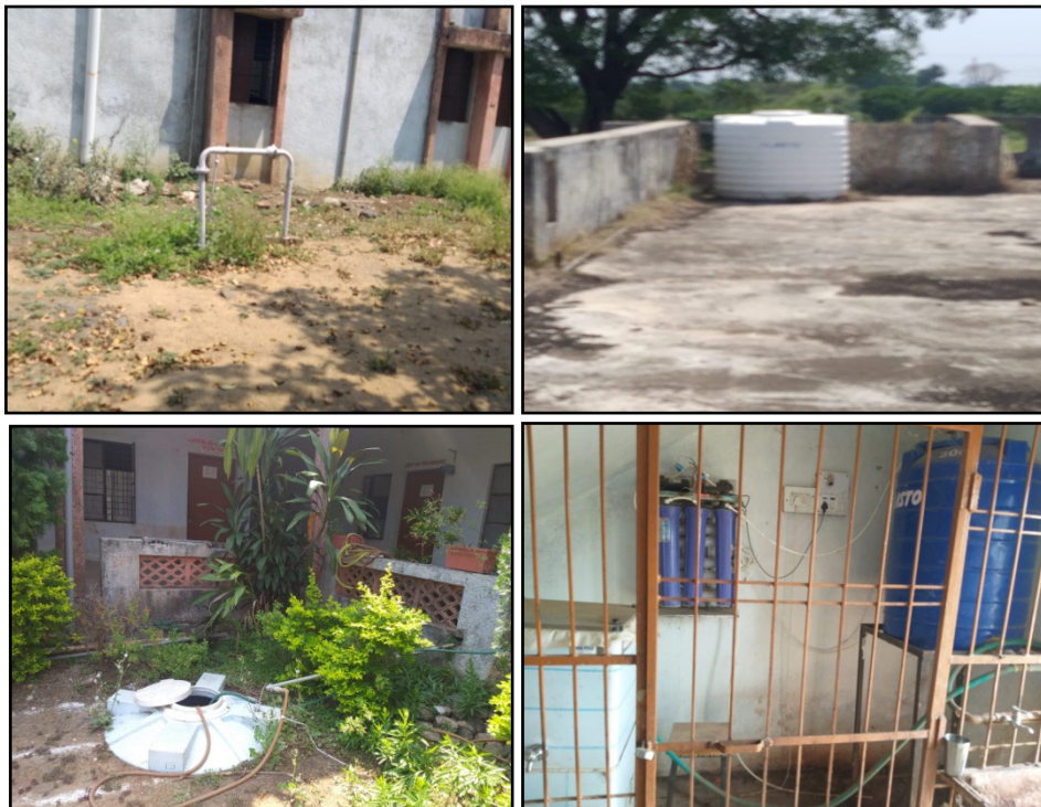
Fig. 3 Bore well, Water Storage Units, Water Cooler and RO Water Purifier System
